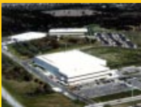
Tokyo Electron Texas, Inc., shown with Tokyo Electron America, Inc.'s head office and parts and training center in the background, produces advanced CLEAN TRACK coater/developers.
