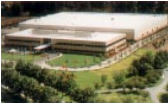
Since building Tokyo Electron Oregon, our first U.S. manufacturing facility, we have added others to ensure timely response to customer demands.
